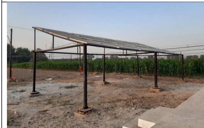
3-PV System for Irrigation
