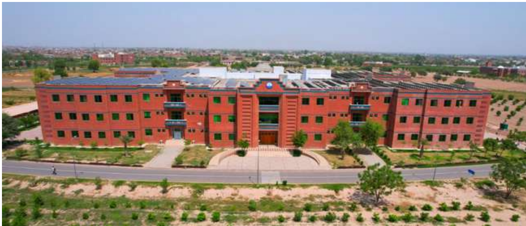
BUILDING IN BLOCK B (ACADEMIC BLOCK) 18335 SQUARE METRE
