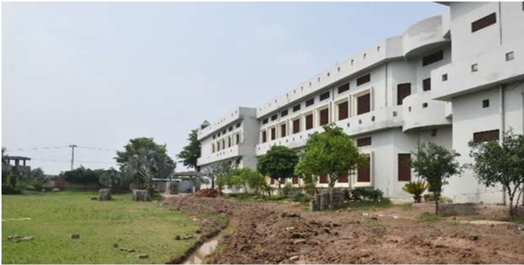
CONCRETE BLOCKS PAVED AT POSTGRADUATE BLOCK (BEFORE)
