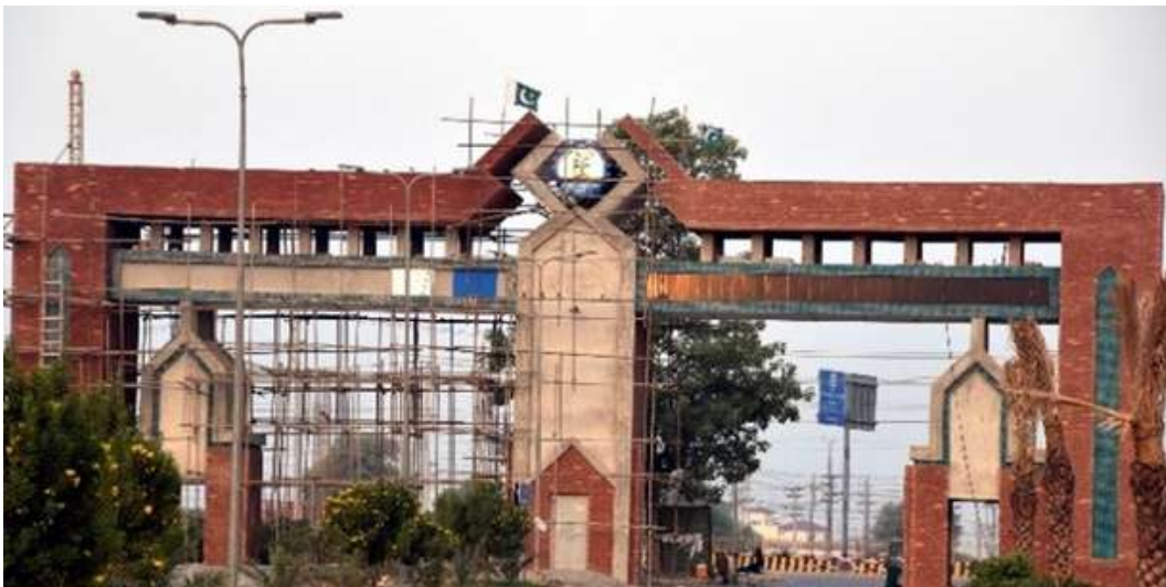
RENOVATION OF UNIVERSITY MAIN ENTRANCE GATE
