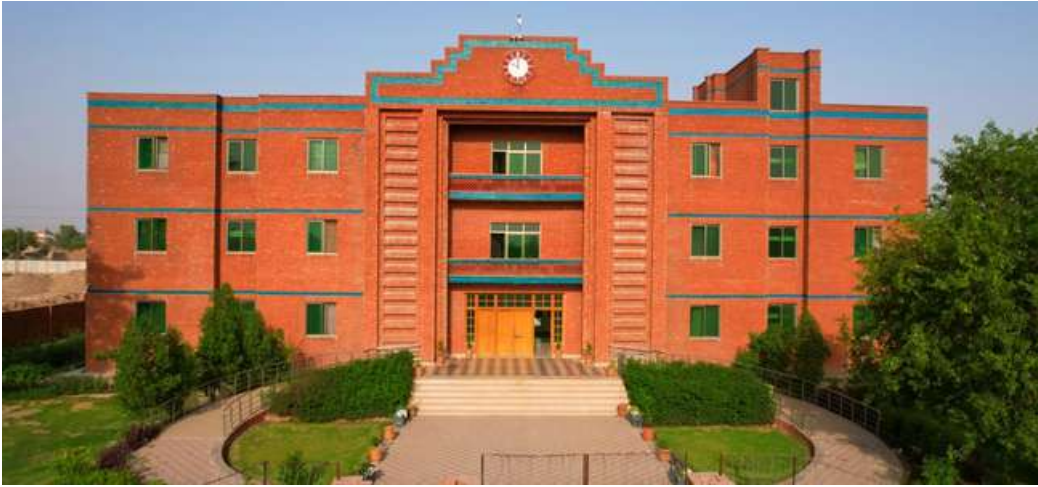
BUILDING IN BLOCK A (GIRLS HOSTEL) 5,825 SQUARE METRE
