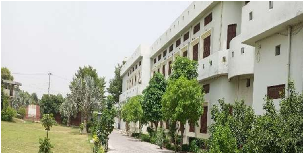
CONCRETE BLOCKS PAVED AT POSTGRADUATE BLOCK (AFTER)
