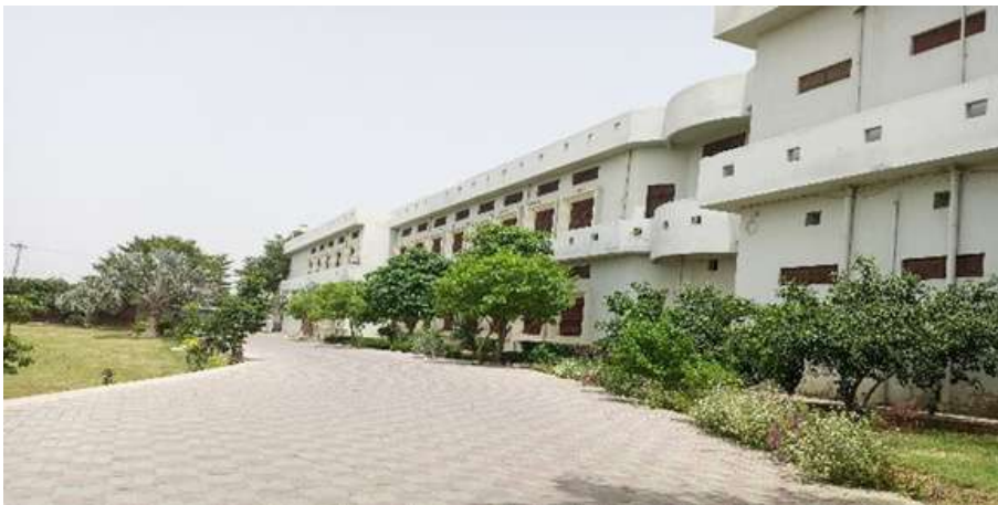
CONCRETE BLOCKS AND LAWN AREA (POST GRADUATE BLOCK)
