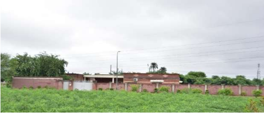
BUILDING IN BLOCK A (VICE CHANCELLOR RESIDENCE) 395 SQUARE METRE
