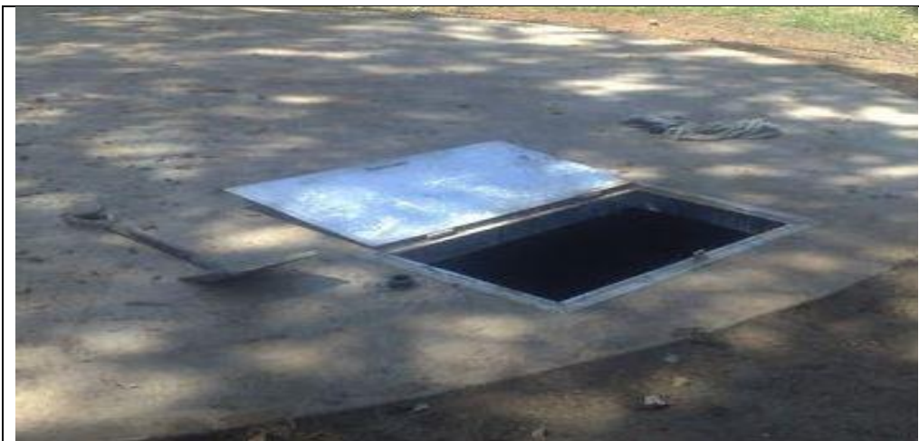
Water Conservation - In Ground Water Tank (Muhammad Nawaz Shareef, University of Agriculture Multan)
