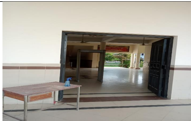
Hand Sanitizer at the entrance of the A Block Building
